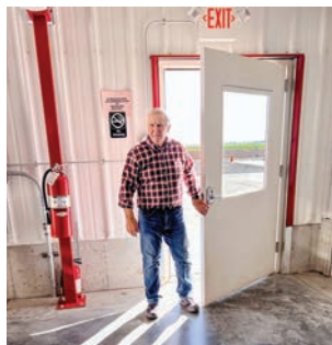
Four-foot wide service doors provide extra room for Russell Patterson and others to pass through.
