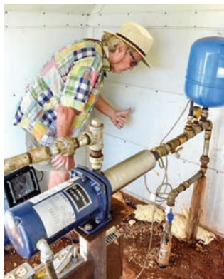
□ A 100-plus-year-old spring-fed reservoir (above) supplies Terry Hodgson's ranch watering system and related fiberglass stock tanks. A pressure-sensitive pumping system in a nearby "well house" (right) feeds all but the highest elevation pastures, which are fed with an additional booster pump.
